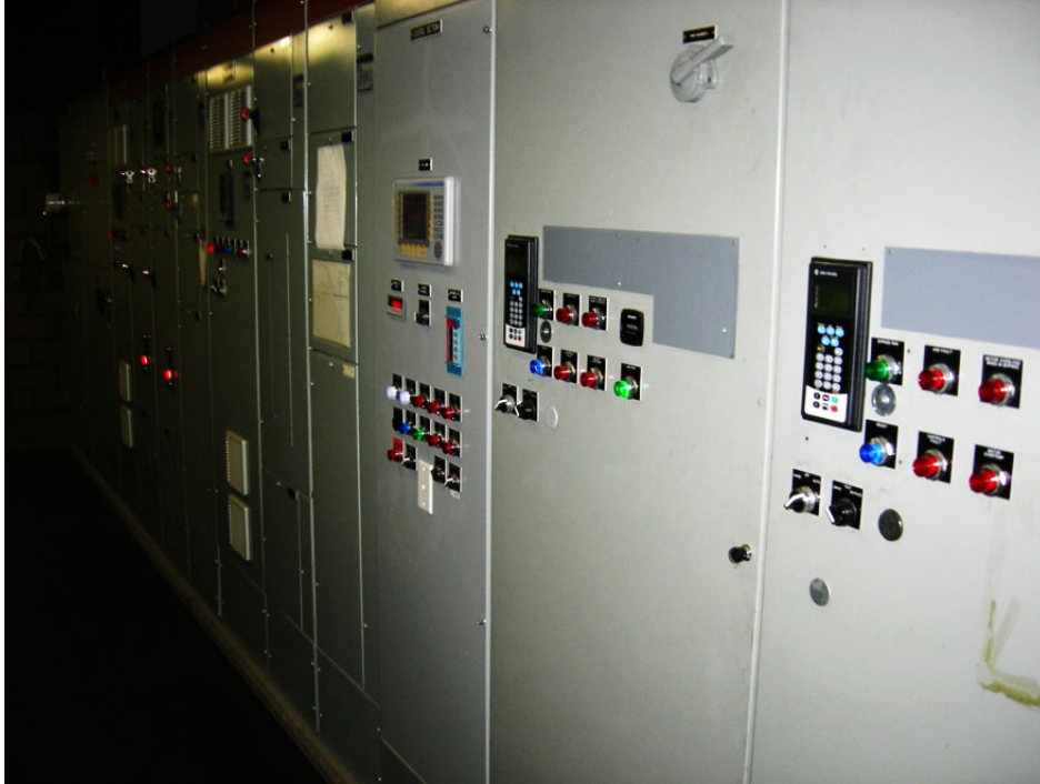
Recycled water treatment facilities
