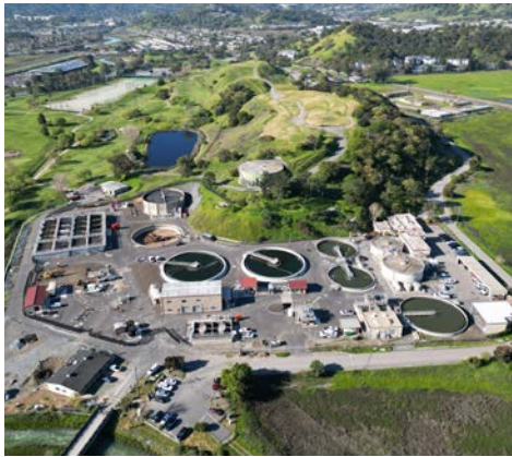
District's Wastewater Treatment Plant — upgrade completed June 2023.
