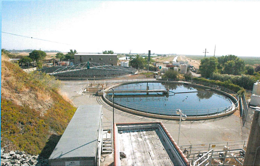
Treatment plant upgrades
