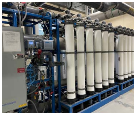
Ultrafiltration membranes for additional recycled water capacity were a major component of the District's $68-million treatment plant upgrade and expansion. 54
