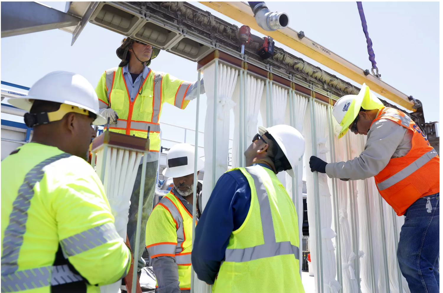
Workers install membrane bioreactors at the Metropolitan Water District's pilot water recycling facility in Carson in 2022. (Christina House / Los Angeles Times)
