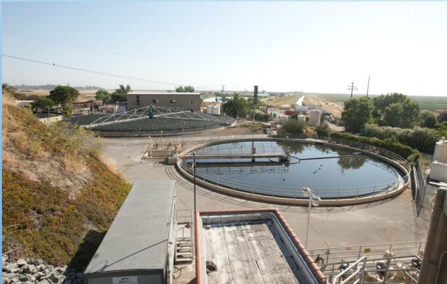
Treatment plant upgrades
