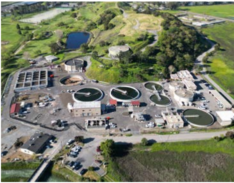
District's Wastewater Treatment Plant — upgrade completed June 2023.
