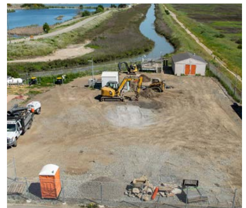
The start of Phase 3 construction.
