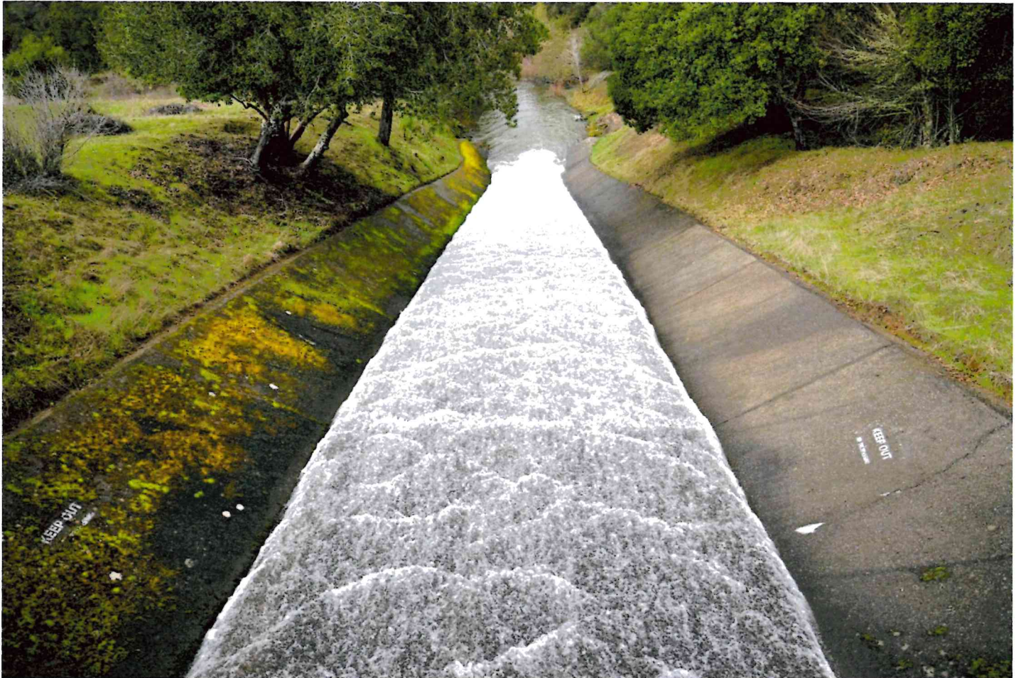
Runoff water flows down the Bon Tempe Reservoir spillway in January in the Mount Tamalpais watershed. The Marin Municipal Water District has seven reservoirs. PHOTOS BY SHERRY LAVARS — MARIN INDEPENDENT JOURNAL
