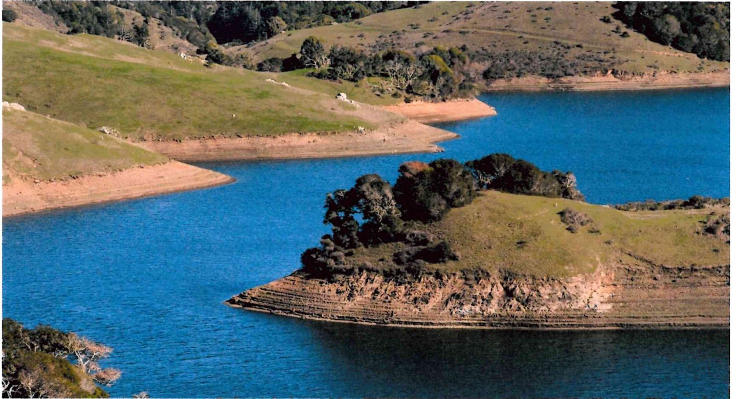
Expansion of the Soulajule reservoir is among the proposals of the Marin Municipal Water District to increase water storage capacity. SHERRY LAVARS — MARIN INDEPENDENT JOURNAL, FILE
