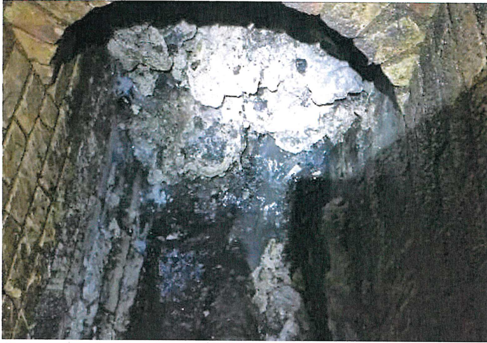
A view of the fatberg that caused a massive clog in the sewer system in 2017 in Whitechapel, London. (Thames Water via AP)
