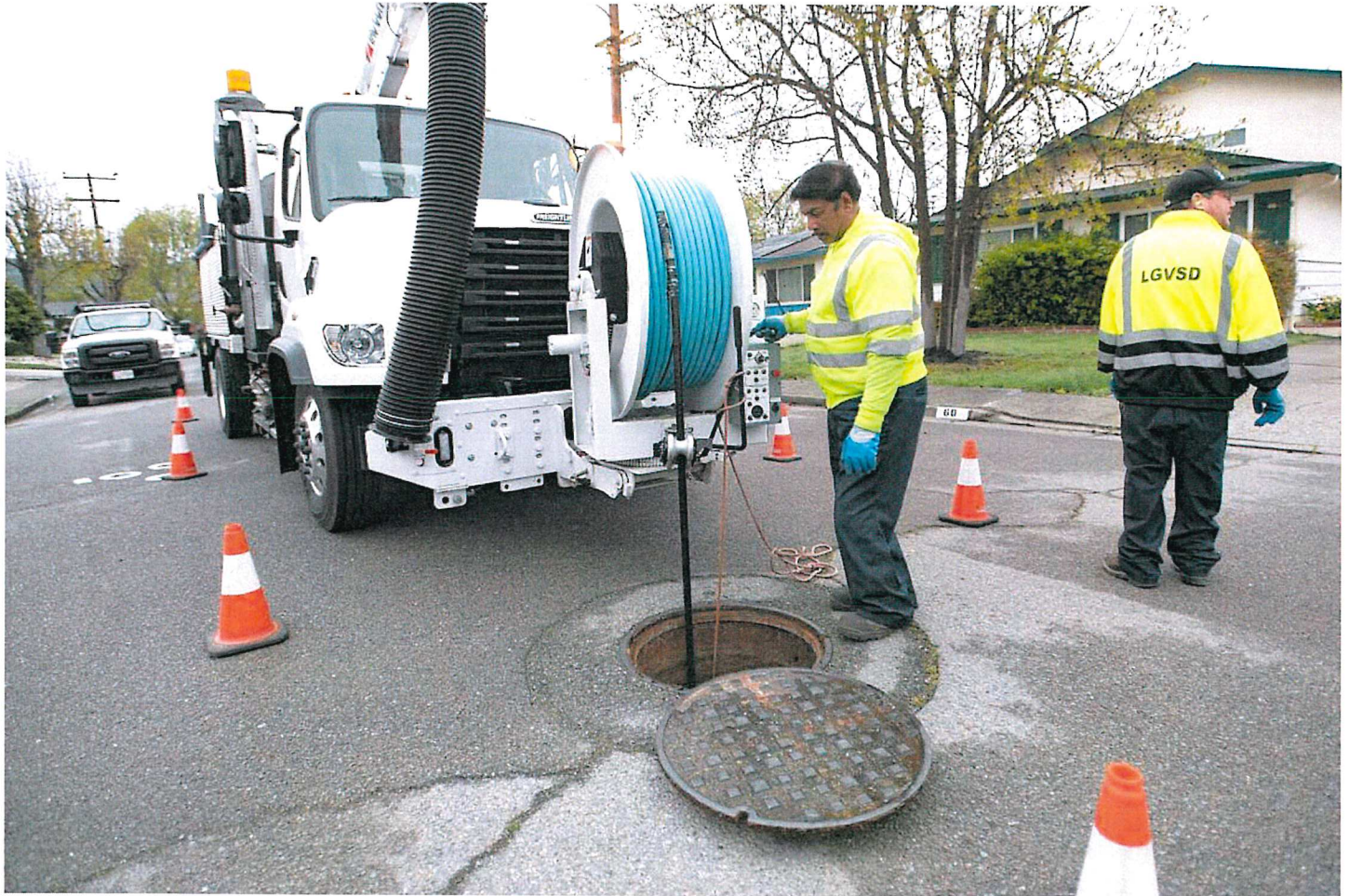
Robert Fernandes (left) and Anthony Asaro of the Las Gallinas Valley Sanitary District show how their crews perform maintenance on sewer lines in San Rafael.
