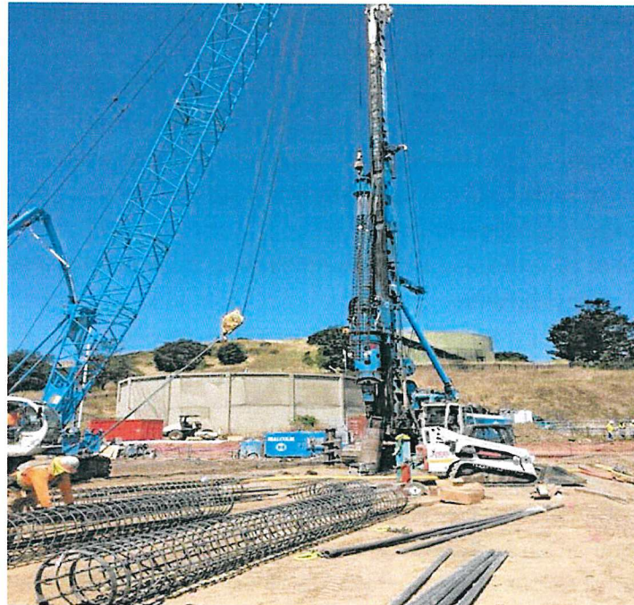
Figure 1. STPURWE Project Caisson Drilling for Aeration Basins in June 2019.
