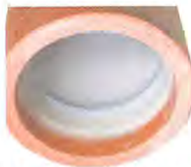
LMK Mainline Sectional Repair
