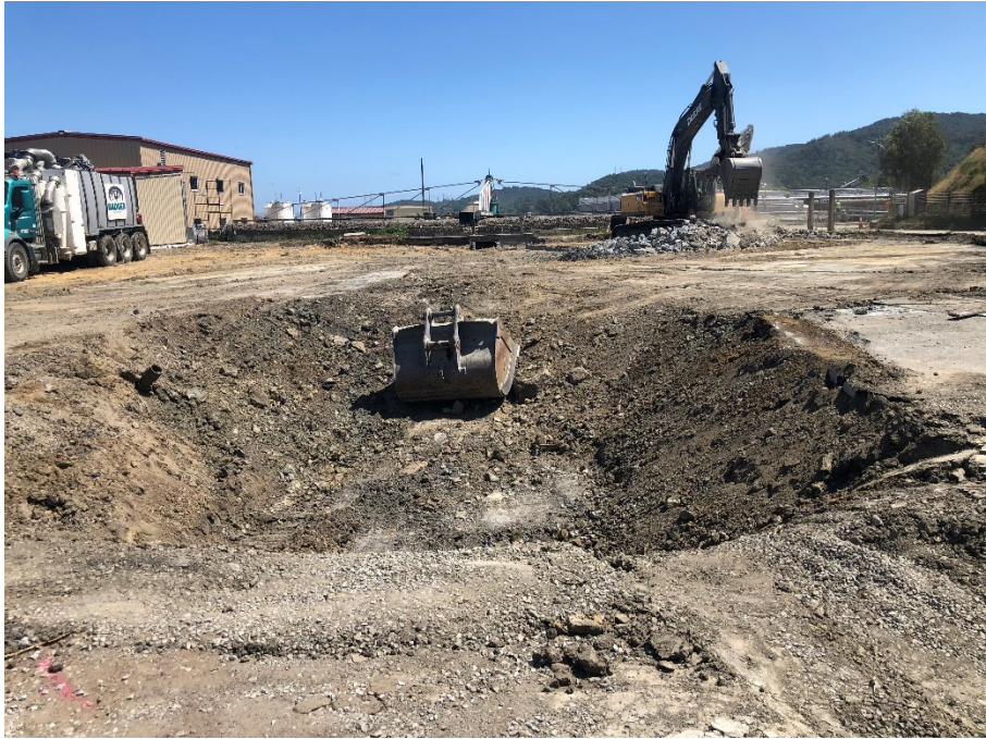
Demolition related to Treatment Plant Upgrade Project
