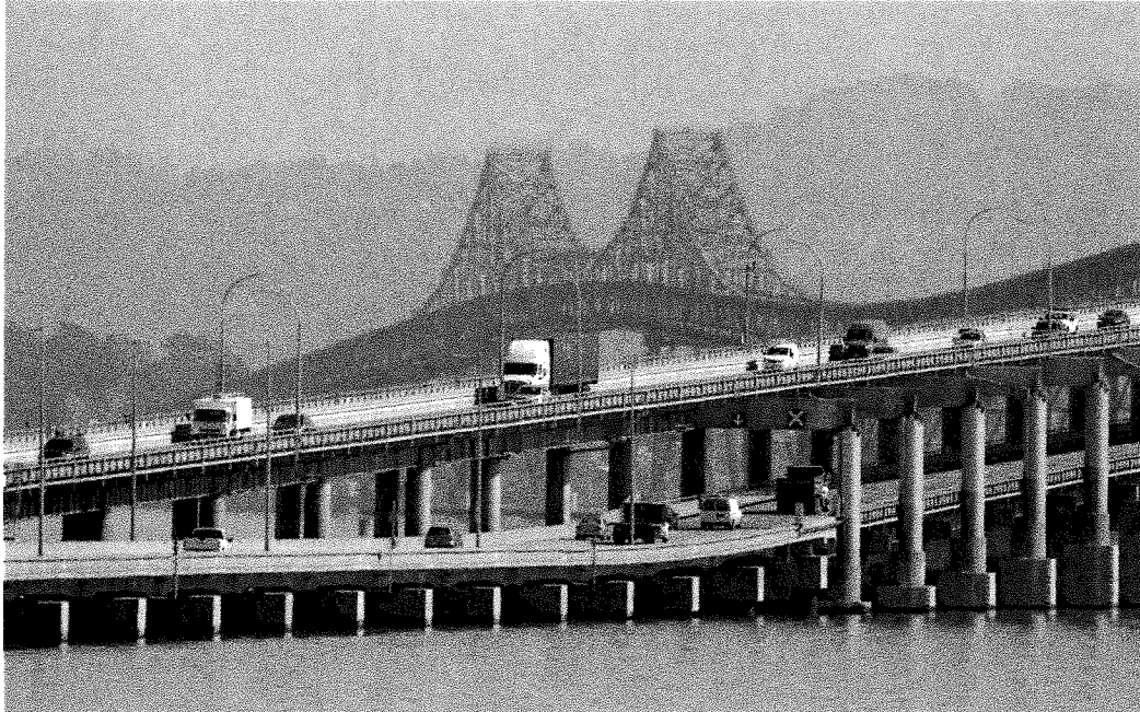
Traffic flows across the Richmond-San Rafael Bridge. The Marin Municipal Water District has considered building a water pipeline across the span.
