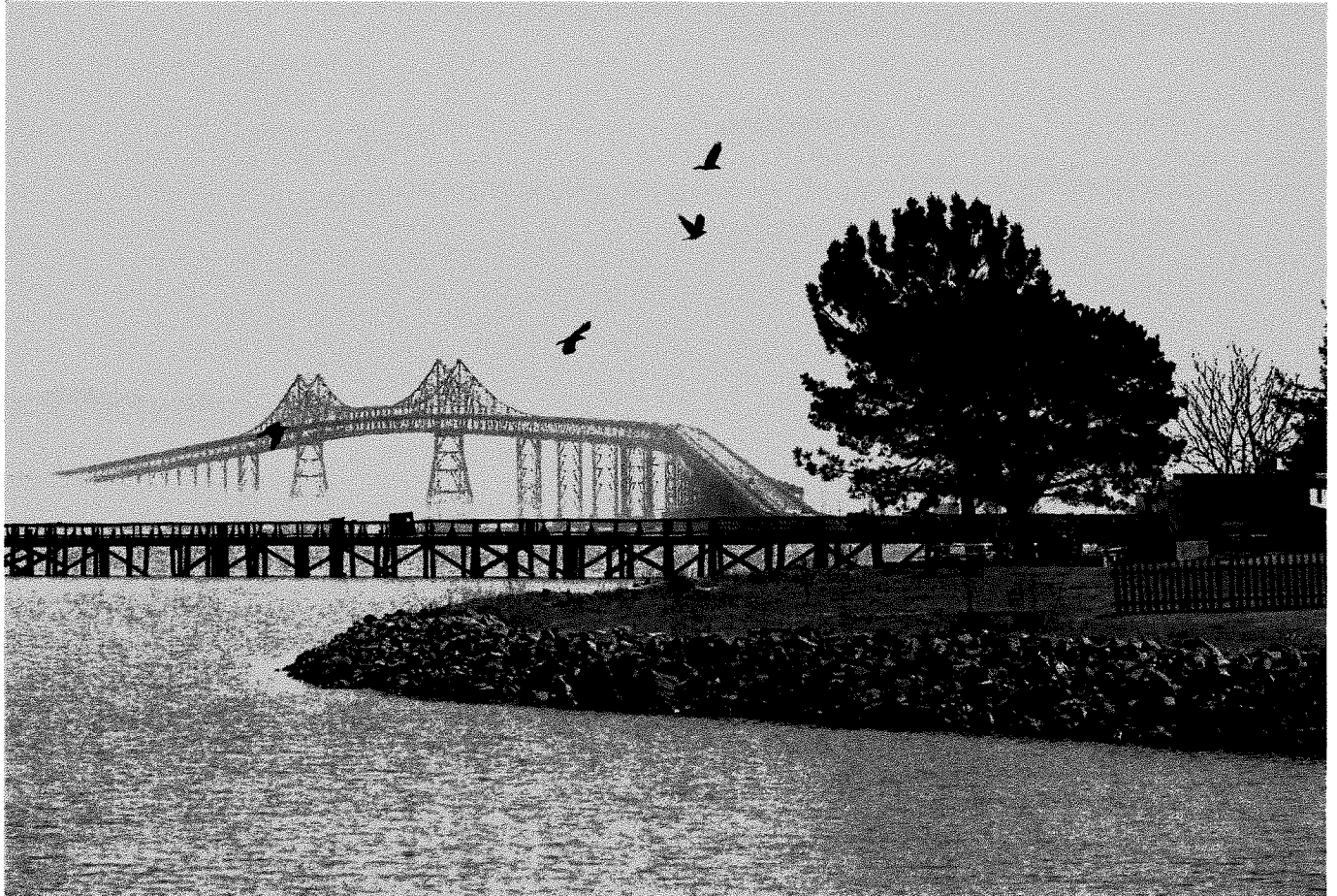
The Marin Municipal Water District has tested desalination near the Marin Rod and Gun Club site a couple of times in the past 30 years. The district launched a study into new water sources after facing potential reservoir depletion from the drought. PHOTOS BY ALAN DEP — MARIN INDEPENDENT JOURNAL, FILE
