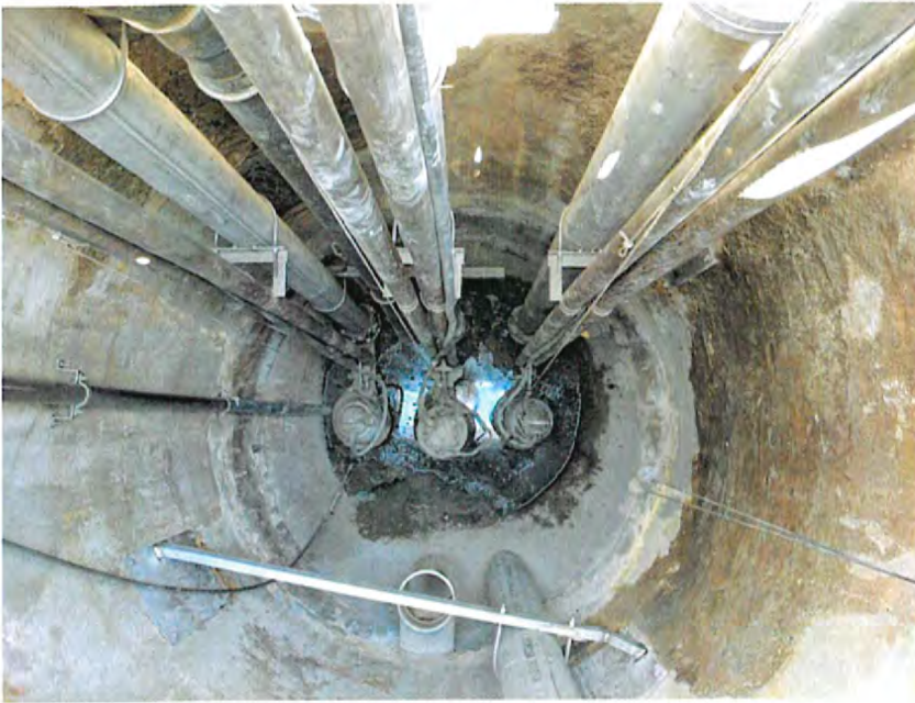
Descanso pump station wet well upgrade project
