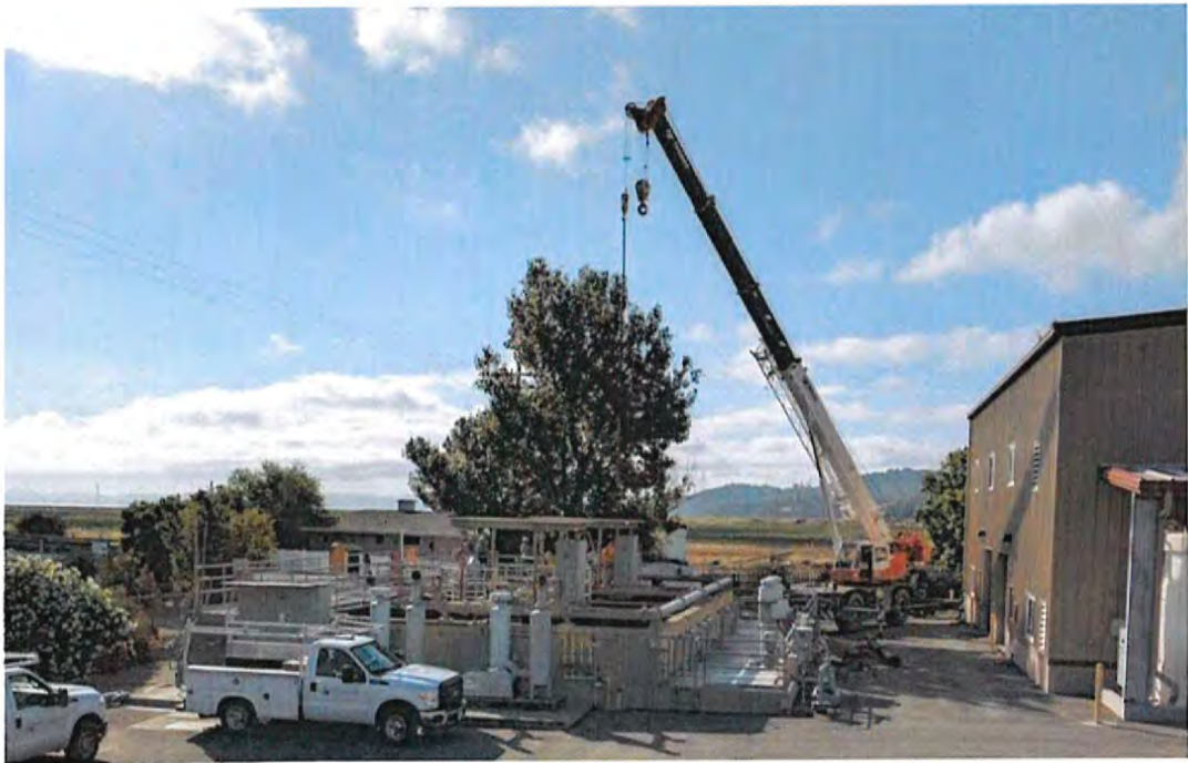
Deep Bed Filter Inlet Valve Replacement Project
