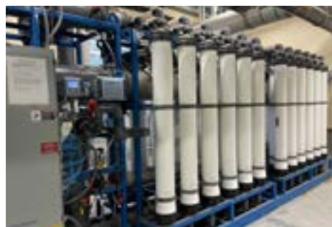
Ultrafiltration membranes for additional recycled water capacity were a major component of the District's $68-million treatment plant upgrade and expansion.
