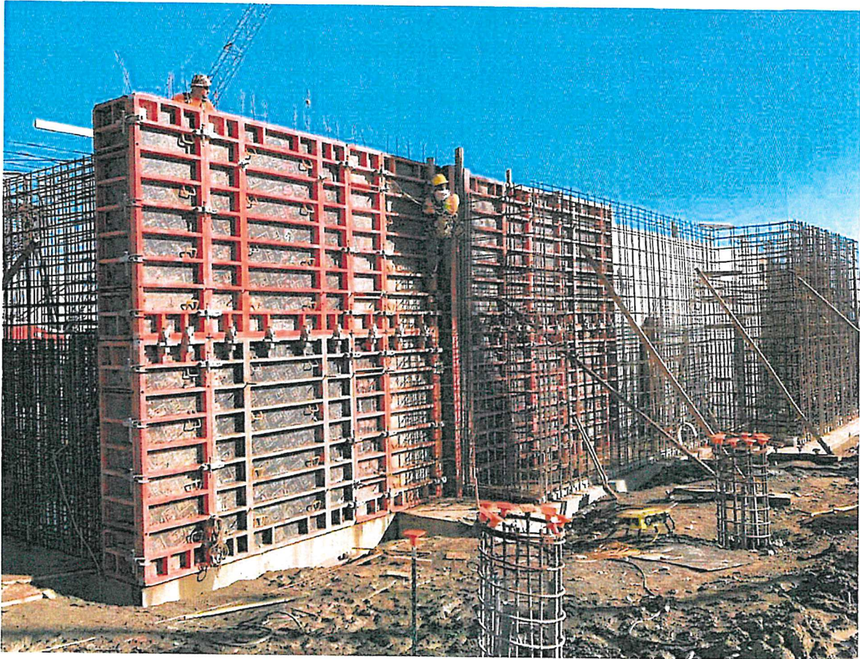
Figure 1. Construction of Aeration Basins. Photo taken on 12/23/2019.
