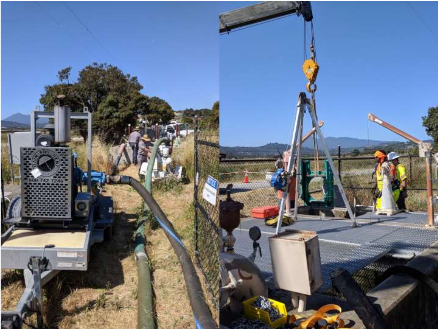
MMWD Recycled Water Facility Pump Station Gate Valve Repair Project
