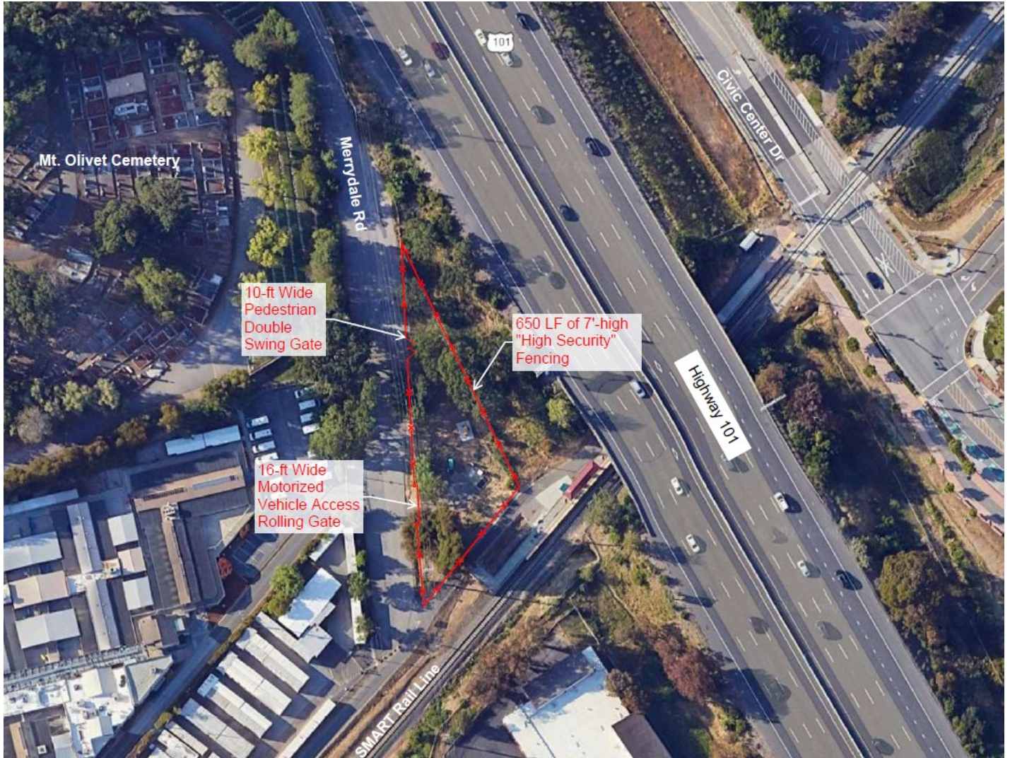
Figure 1. Rafael Meadows Pump Station Approximate Boundary
