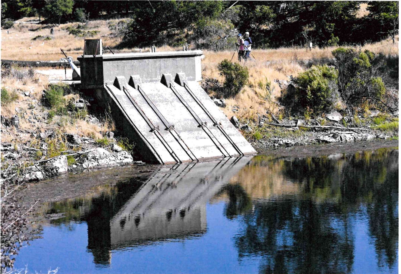
Hikers approach a concrete structure with gate valves at Lake Lagunitas in the Mount Tamalpais watershed. The lake is a Marin Municipal Water District reservoir. SHERRY LAVARS — MARIN INDEPENDENT JOURNAL
