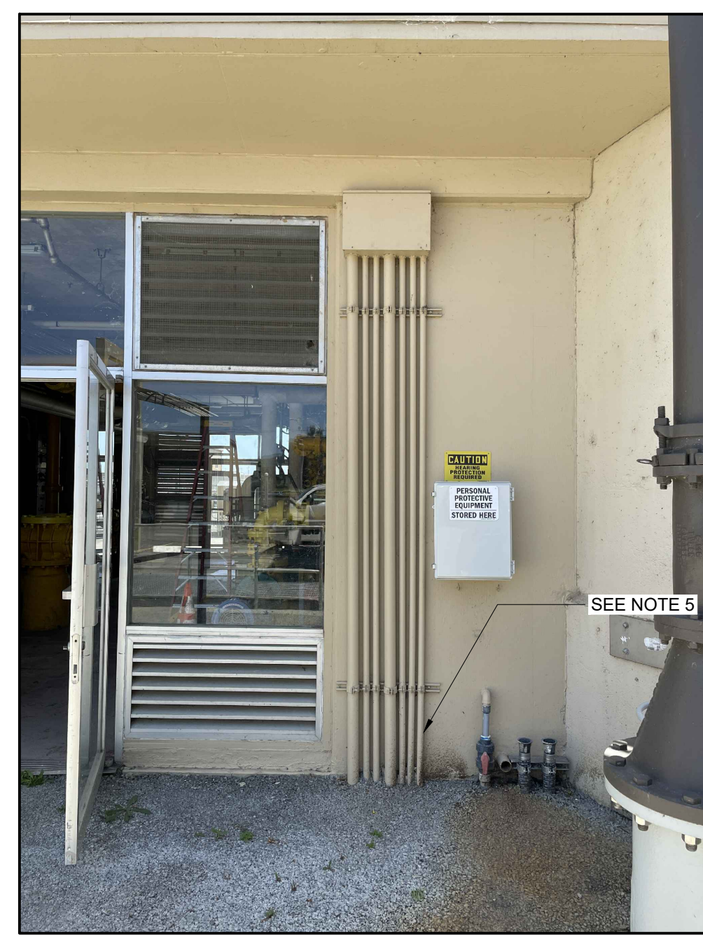
CONDUIT STUB-UP SEALS (NOTE 5) SECTION 1 NTS E04
