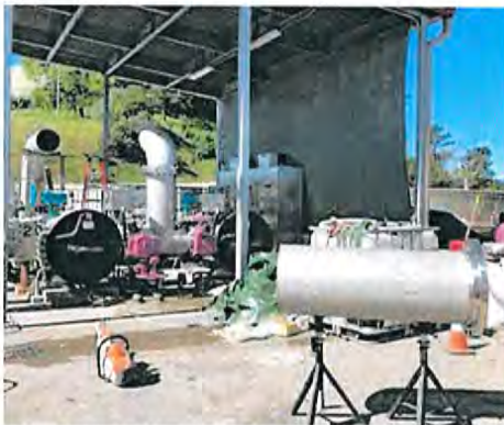
Fabricating new stainless steel pipework at the UV building.
