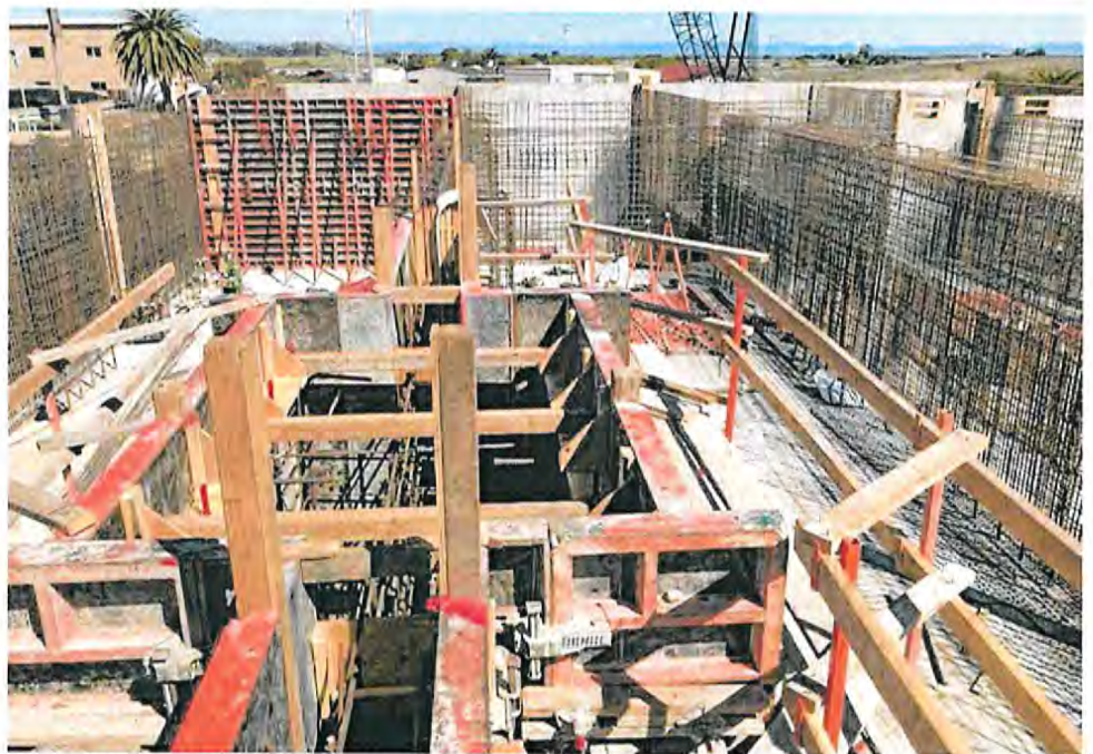
Aeration basin interior walls formwork and rebar.
