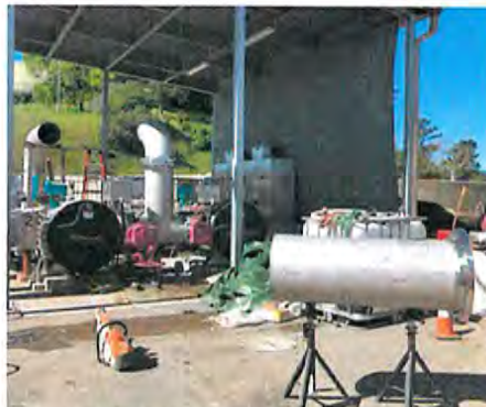
Fabricating new stainless steel pipework at the UV building.
