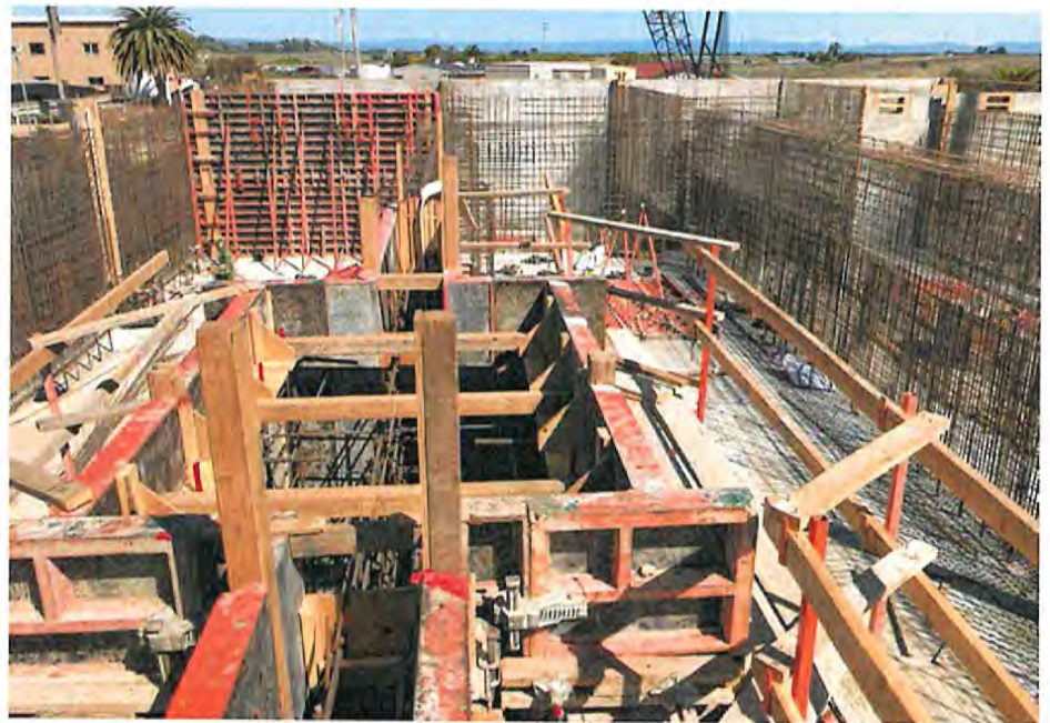
Aeration basin interior walls formwork and rebar.
