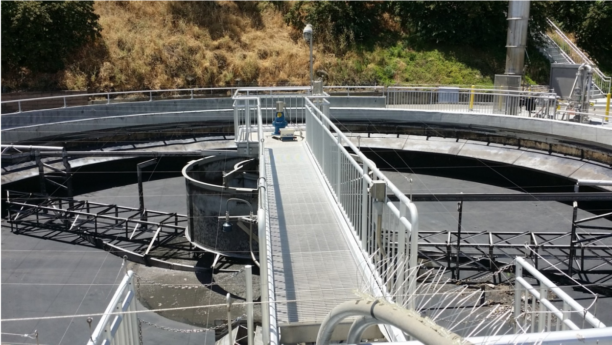
Primary Clarifier #3 Drained, Inspected and Stamford Baffles Removed
