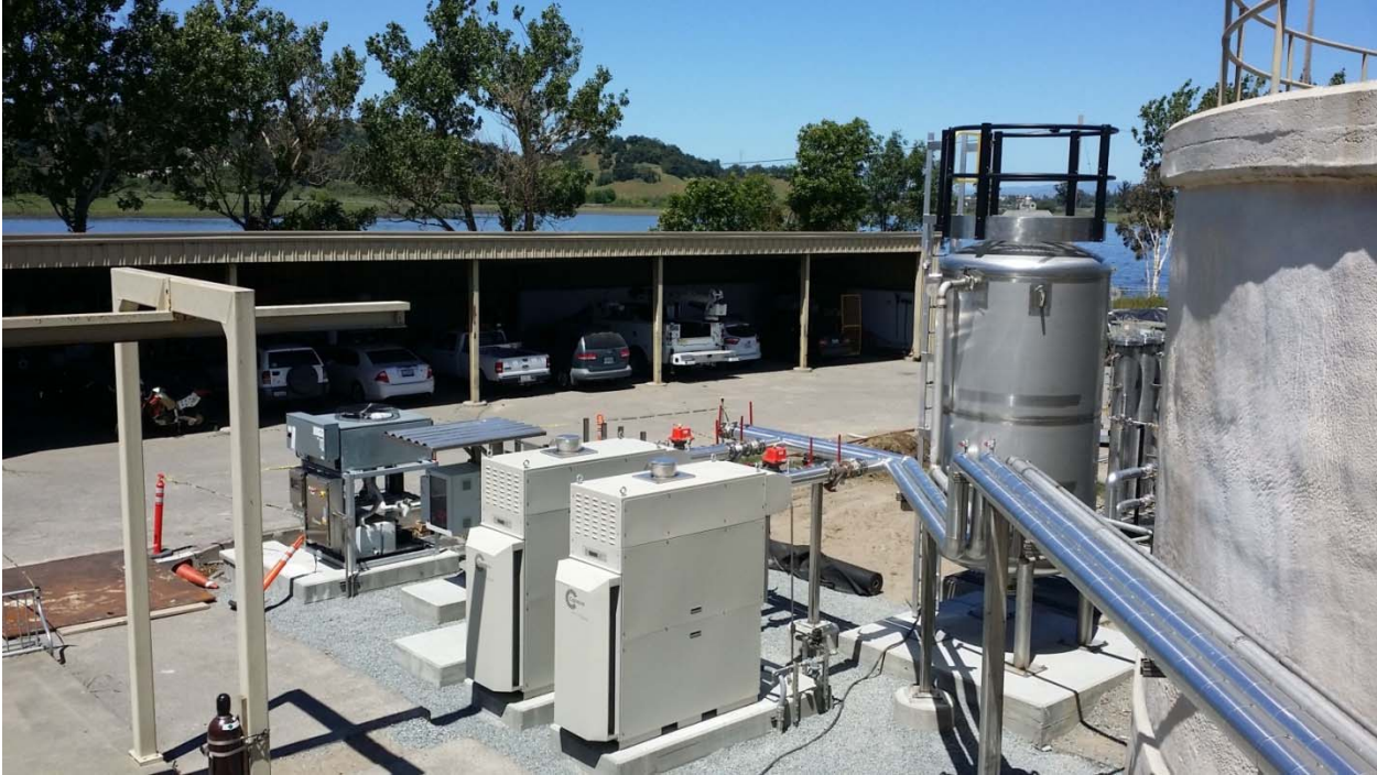
BERS Project Ready for May 9, 2016 Start Up
