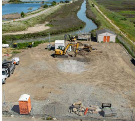
The start of Phase 3 construction.
