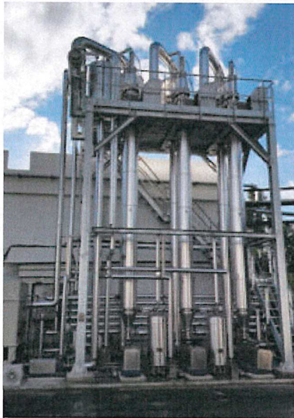
HRS energy-efficient multieffect digestate concentration system
