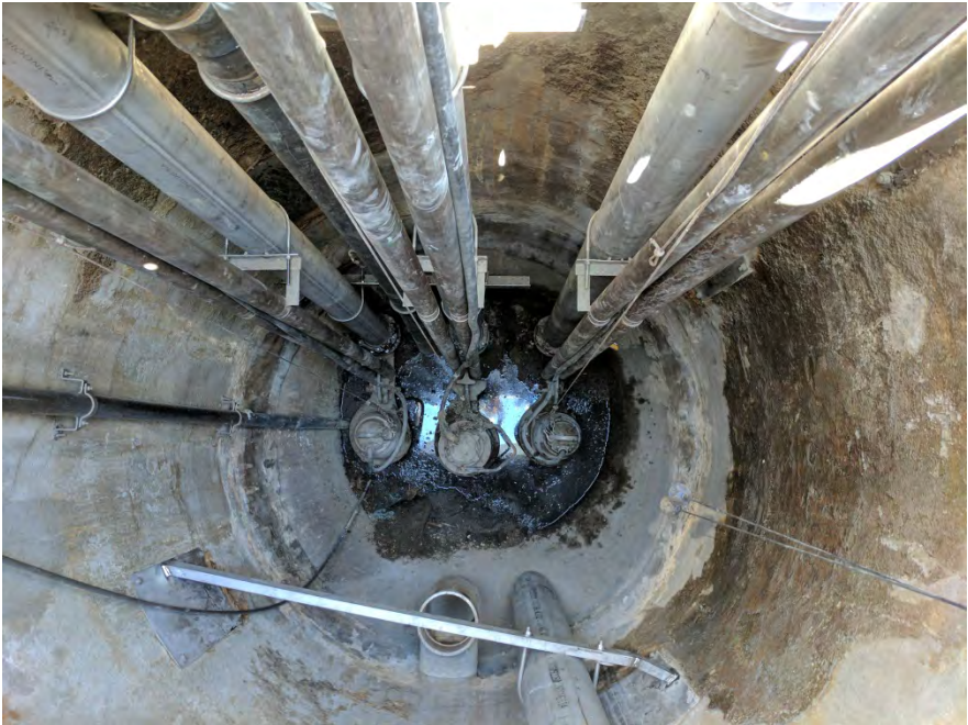
Descanso pump station wet well upgrade project
